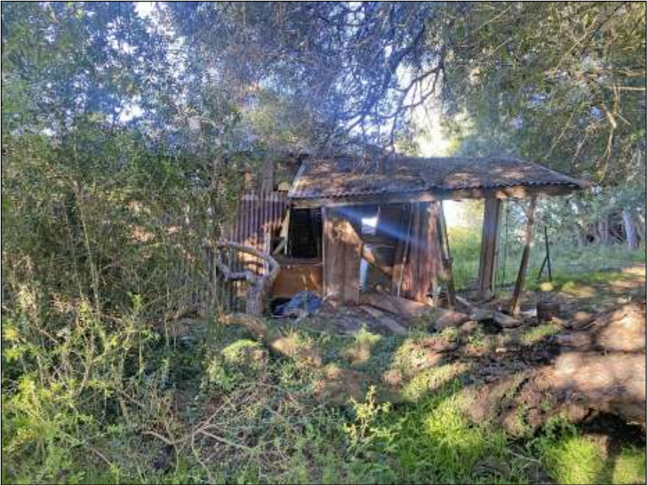
Front view of Dabinett home taken in August 2025. The same place from which the c1873 photo was taken. Note that half of the verandah has collapsed and part of the front wall has fallen down. Yet the original vertical timbers remain visible on this wall. (K Cordina)
